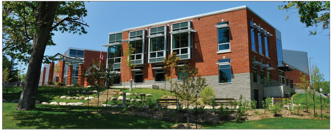
PHOTO CREDIT ENERMODAL ENGINEERING
