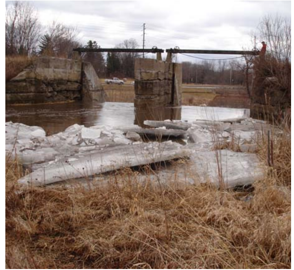
In-line Structure on Cobourg Creek
