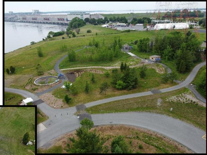
Bioswale features located through the trail system were designed to contribute to runoff reduction, erosion control and improved infiltration, achieving benefits on the water quality and water balance of the site.
