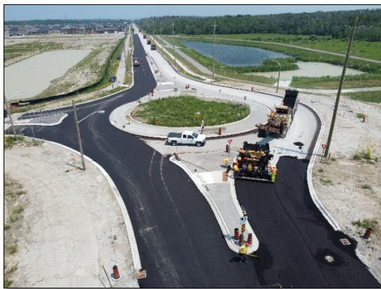
Roundabout at 6 th Line & Webster Blvd., Innisfil ON
